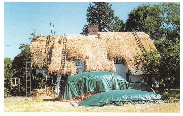
Fig 12 Thatching long straw to a basecoat
