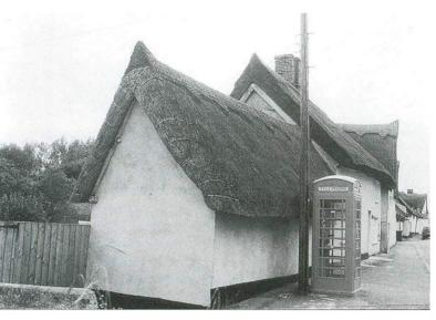
Fig 4 This long straw roof in Suffolk, with its distinctive wrapped and cut gables, is typical of the steep pitches found in east Anglia. (Photograph copyright @ Rural Development Commission)
