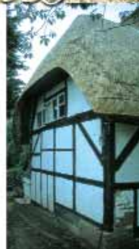
Above: Long straw verge finished with cross-rods, Cheriton.
