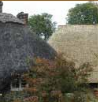
Above: Two distinct thatching styles showing weathered combed wheat with a block patterned ridge and new longstraw on right with a twisted knot ridge, Ibthorpe.
