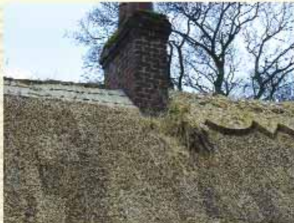
Above: Block patterned ridge in straw on water reed, Cowleaze Cottages, Longparish.
