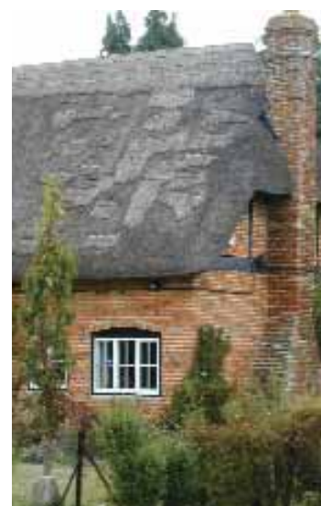
Below: A traditional patch repair will extend the life of the thatch, St Mary Bourne.
