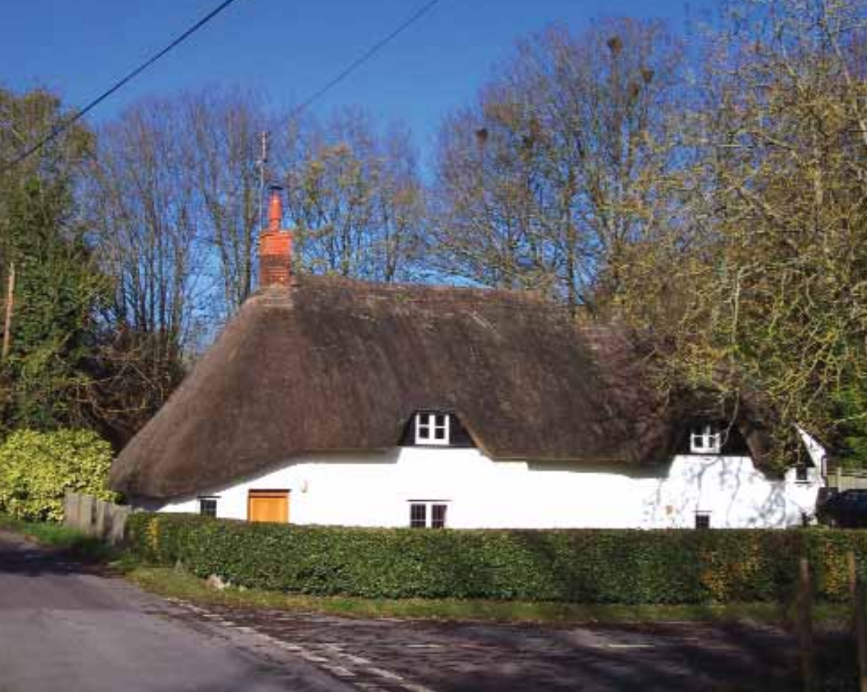
Left: Combination thatch, Bridge Cottage at Quarley
