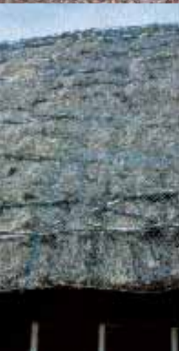
Above top: Excessive moss cover will hold moisture against the thatch, Longstock.
