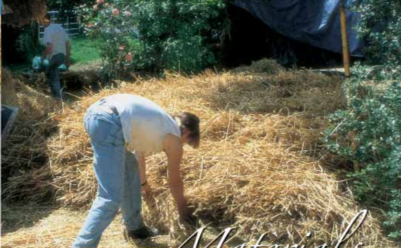
Right: "Good thatch is made on the ground" yealming at Poplar Farm, Longstock.
